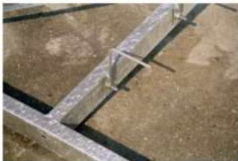
Typical Flex Anchor showing Degrees of Freedom
